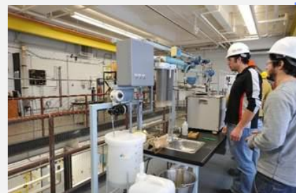
Engineering Operations (FM Hard Services):
